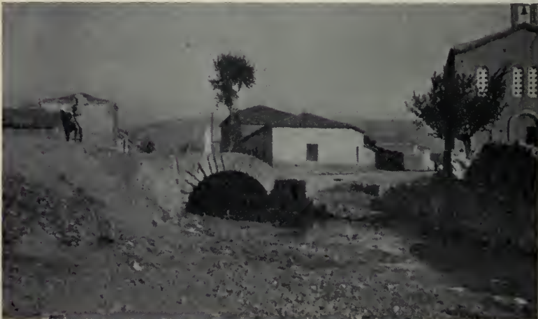
AN OUTFALL SEWER NEAR DANIELS' CHURCH, ATHENS
